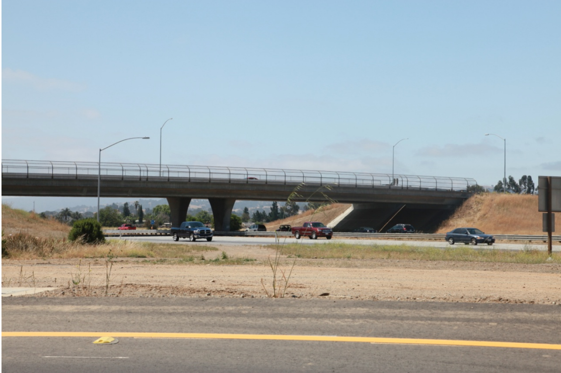
Figure 2. Tennant Avenue Bridge shown from the southwest.
