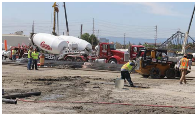
Above: Start of concrete works for the stadium foundations.
